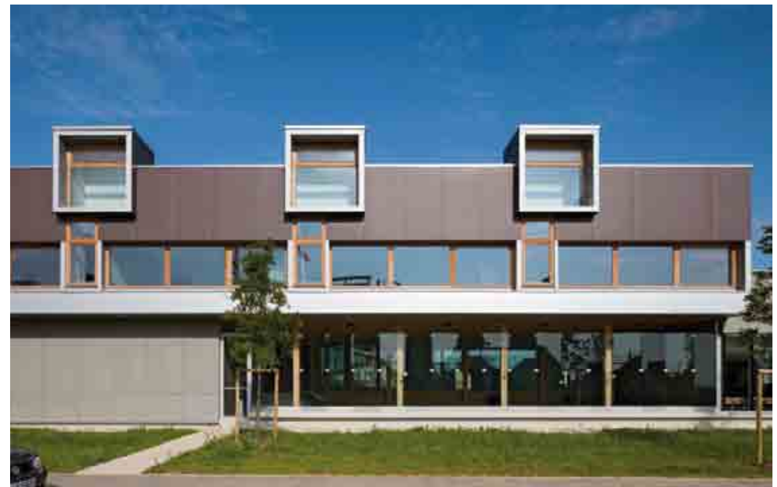
Fibre cement panels in three different colours clad the street façade of the primary school.
